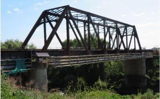
The present bridge over the Hunter River. A train driver noticed that steel work in the top section of the bridge had cracked.
