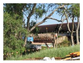
Steel barriers to prevent further slippage of earthworks at the subway. Beautification work will be undertaken on Completion.
