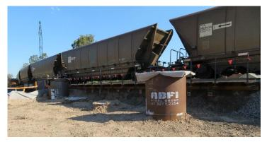
Pylons in place west of the subway. These are double pylons with an interior core pylon for safety if a train was to come off the tracks.
