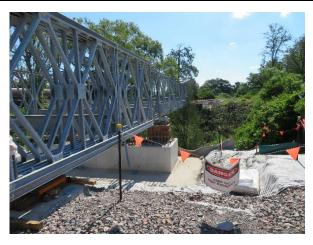
This photo shows the bridge out over Muscle Creek heading towards the abutment already formed on the other side. At the present time all access to the other side is through the caravan park. This will not be possible when the pylons and abutments are being constructed for the permanent bridge. All the concrete and steel for the huge sections will be trucked in through the site in Lower Williams Street.
