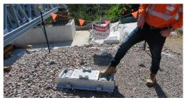
One of the bearings on which the bridge rolls. One under bridge behind on abutment behind flag.
