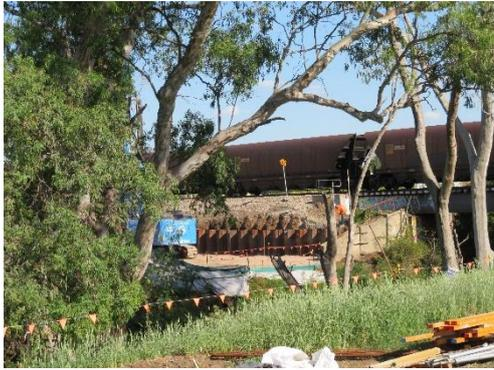
Steel barriers to prevent further slippage of earthworks at the subway. Beautification work will be undertaken on Completion.
