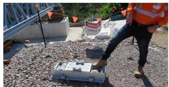
One of the bearings on which the bridge rolls. One under bridge behind on abutment behind flag.
