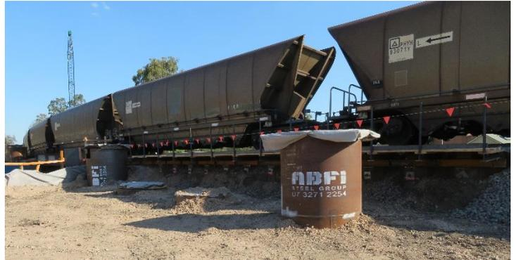
Pylons in place west of the subway. These are double pylons with an interior core pylon for safety if a train was to come off the tracks.
