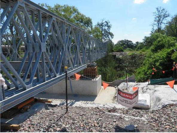
This photo shows the bridge out over Muscle Creek heading towards the abutment already formed on the other side. At the present time all access to the other side is through the caravan park. This will not be possible when the pylons and abutments are being constructed for the permanent bridge. All the concrete and steel for the huge sections will be trucked in through the site in Lower Williams Street.
