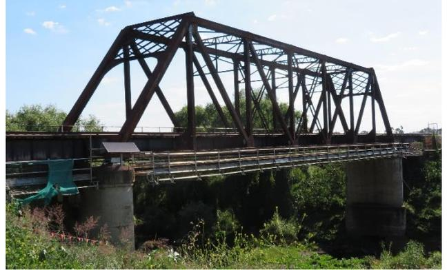
The present bridge over the Hunter River. A train driver noticed that steel work in the top section of the bridge had cracked.
