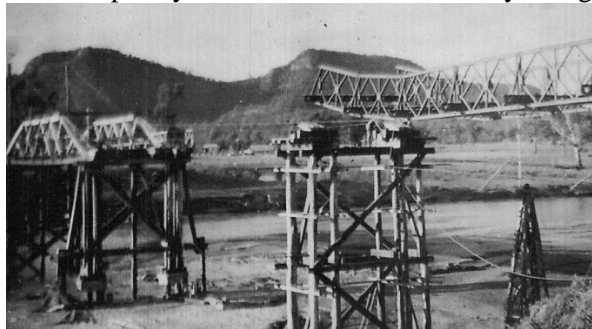
Bailey Bridge being constructed MSL&FHS photo D1331
