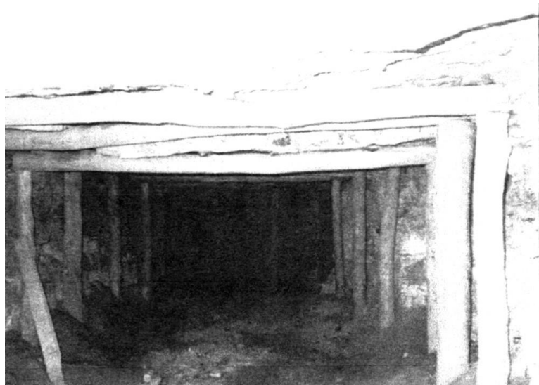
The Bayliss Tunnel
