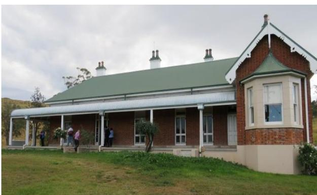
The historic Bengalla Homestead with the new bull nosed corrugated iron verandah. When the house was built the original roof was of cedar shingles. The original plaster which was beyond repair has been replaced using the same method as when the house was originally built.
